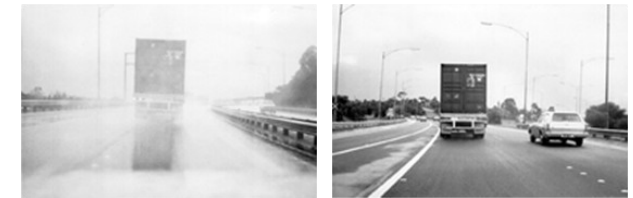
Same truck, same weather but different road surfaces. The surface on the right is an open graded asphalt.
