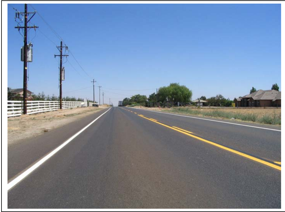
Photograph 2 shows the appearance of a treated road in the County of Merced, California in good profile.
