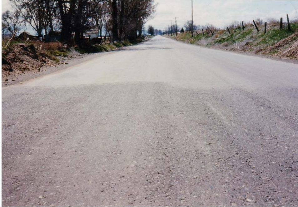
Photograph 1 shows the tightening and densifying effect of a rejuvenator treated pavement. (State of Idaho)
