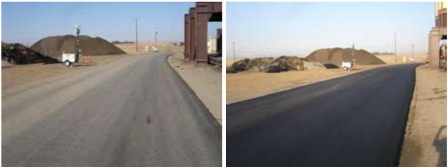
**Figure 4.** Completed haul road at the hot plant and haul road one month later after truck traffic.
