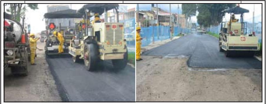
**Figure 3.** *Placement procedure of asphalt mixes*
