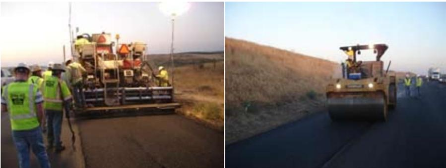
**Figure 6.** Placement and compaction of Astec Double Barrel System test section.
