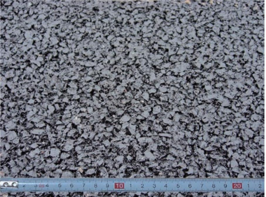
**Figure 7.** *Surface of Porous Rubber-Asphalt in Prague after its paving (scale in millimetres)*
