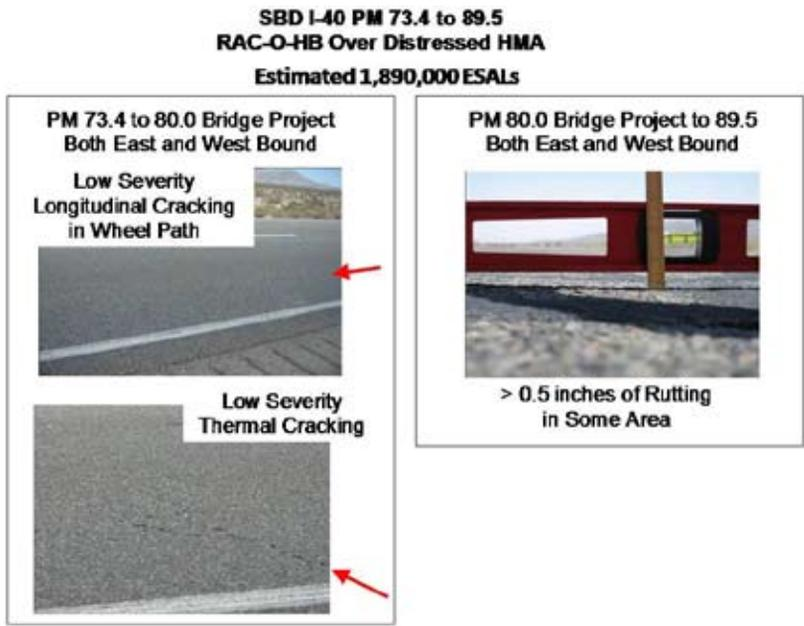
**Figure 8.** Typical condition of SBD-40 PM 73.4-89 after 5 years
