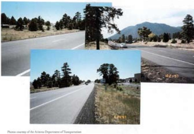
**Illustration 2.** Interstate 40 concrete pavement seven years after overlay with asphalt-rubber mixes
