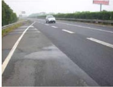
**Fig6.** Pavement permeability performance after raining of Ninggao expressway AR-OGFC overlay (two years after open to traffic)
