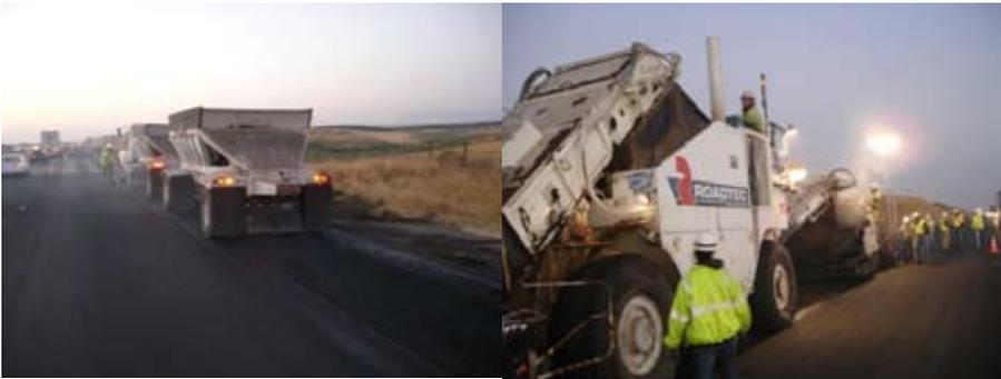
**Figure 5.** Placement of Astec Double Barrel System test section.
