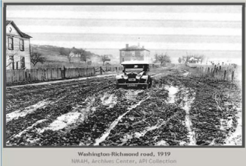
**Figure 2.** *Effect of too much water in the roadway*
