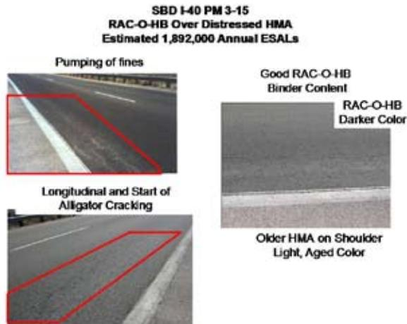
**Figure 7.** Typical condition of SBD-40 PM 3-15 after 5 years
