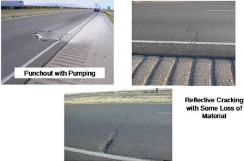
**Figure 5.** Typical condition of FRE-5 after 7 years
