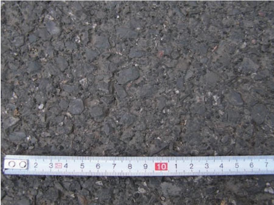
**Figure 6.** *The rubber particles on the pavement surface trafficking for a period of a year (scale in millimetres)*
