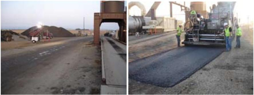
**Figure 3.** Existing haul road at hot plant and placement of test section.
