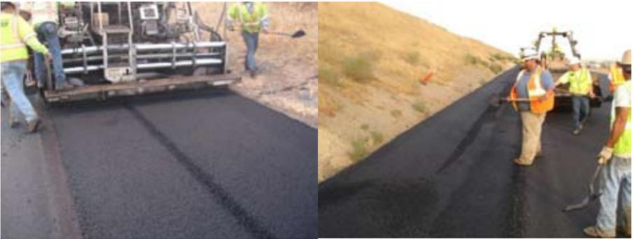
**Figure 8.** *Problems during placement of Evotherm/Astec test section.*
