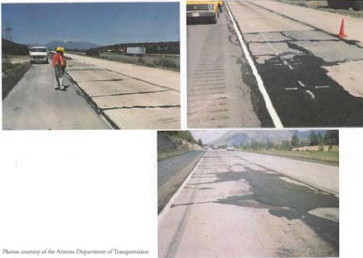
**Illustration 1.** Interstate 40 concrete pavement before overlay with asphalt-rubber mixes
