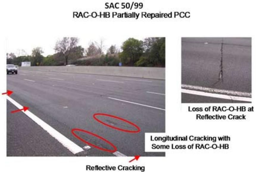
**Figure 4.** Typical condition of SAC 50/99 project after 7 years
