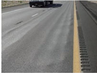
**Figure 2.** *An Example of Failed Project (I-40 West Bound ADOT #3, June 2005)*
