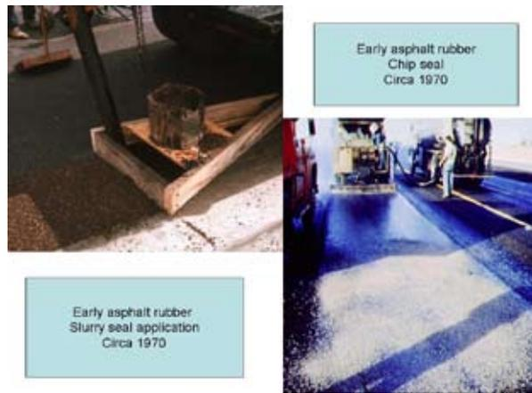
**Figure 2.** *Asphalt-rubber applied as a slurry seal*
