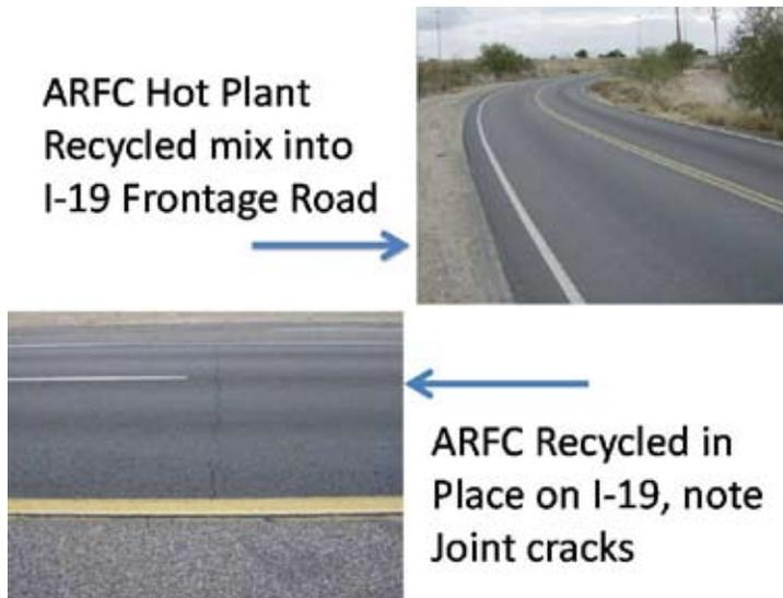
**Figure 17.** *Recycled ARFC pavement*
