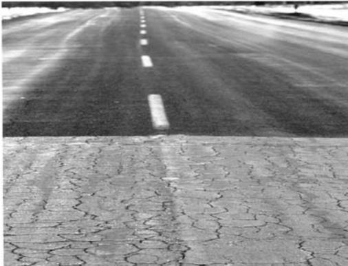
**Figure 4.** *Asphalt-rubber chip seal applied to badly cracked pavement, circa 1972*
