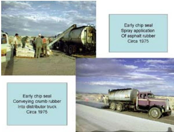
**Figure 3.** *Asphalt-rubber chip seal*
