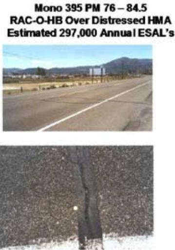
**Figure 6.** Typical condition of Mono 395 after 7 years
