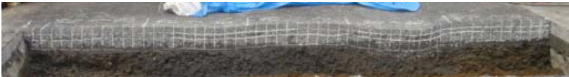
Photo 3 : View of open-cut cross section
