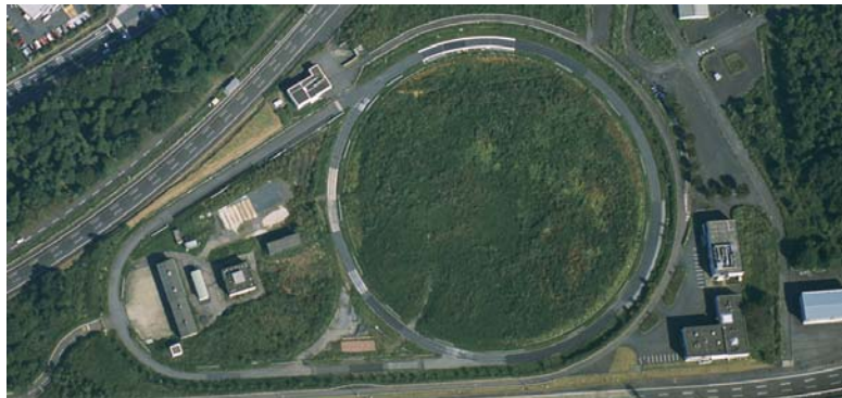
Photo 1 : Pavement Test Field
