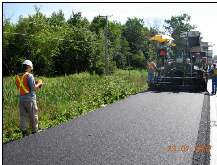
Figure 6: Position for taking temperature measurements behind a paver
