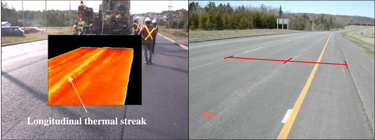
Figure 4: Longitudinal thermal streaks and cracking, usually occurring at centre of the strip
