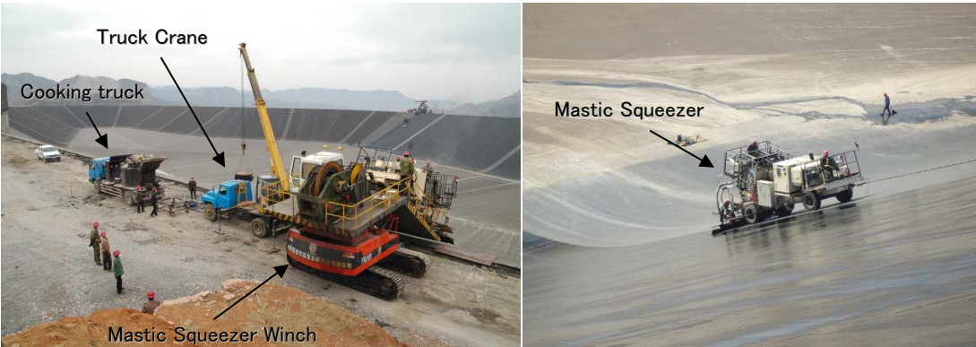
Photograph 4: The construction machine formation for the seal coat
