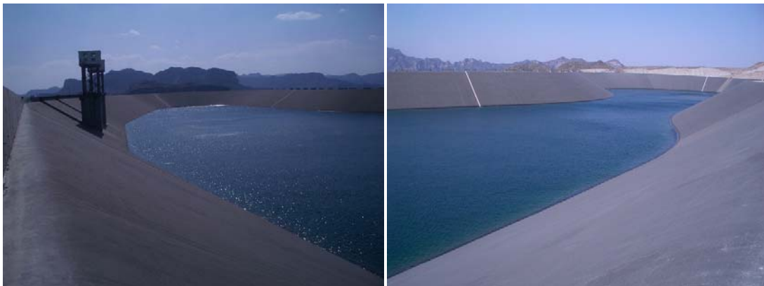
Photograph 5: The completed upper reservoir under impound water condition
