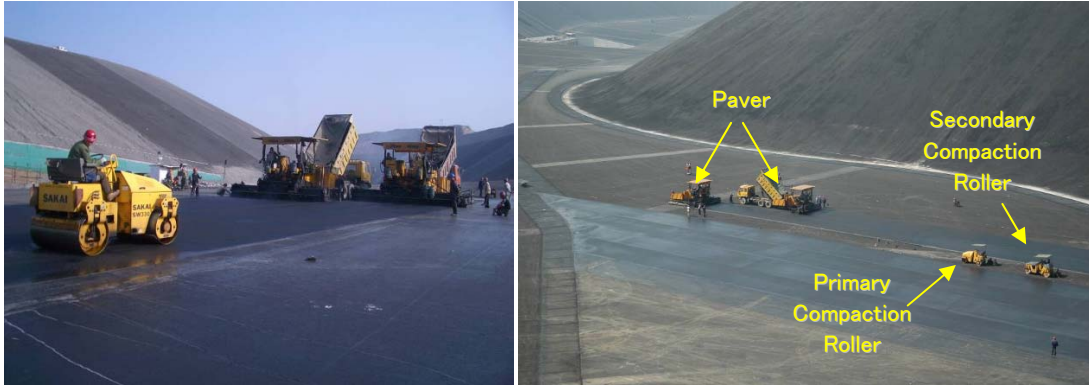
Photograph 2: The construction machine formation in the reservoir bottom
