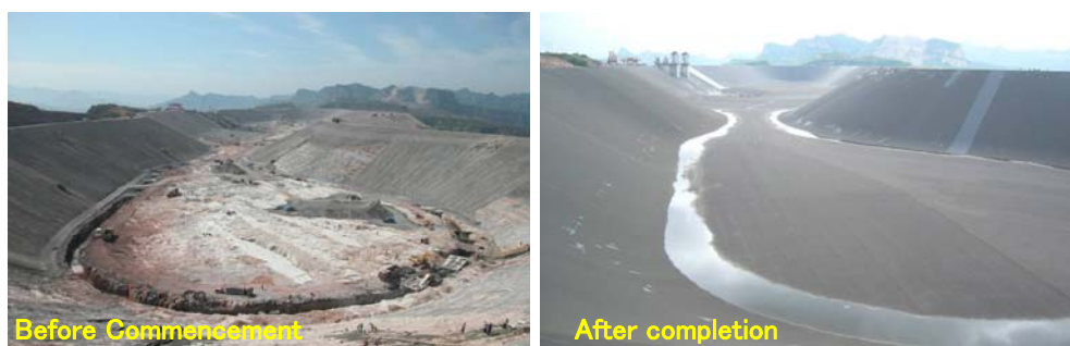
Photograph 1: The full view from north of the upper reservoir
