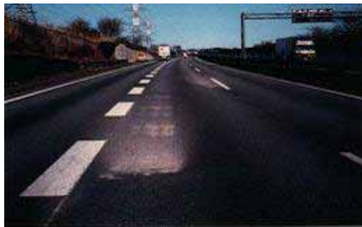
Picture2: Phenomenon of pumping damage
