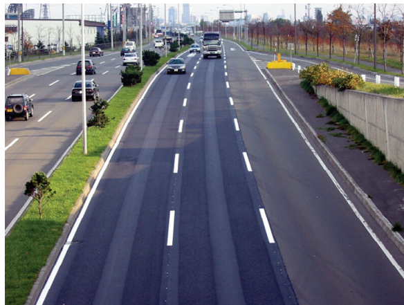
Photo 4 : Rutting Resistant Pavement
