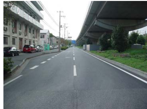
Photo 3: Scene of Test Pavement Site (Two years after)
