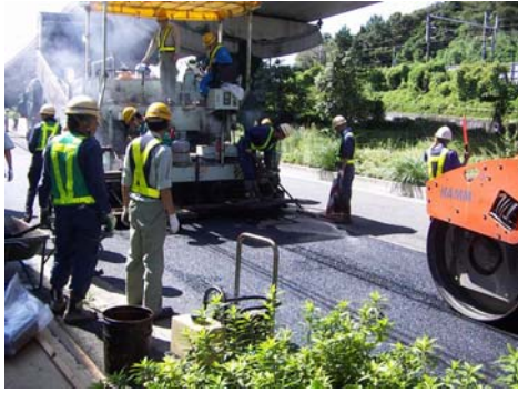
Photo 2: On-site construction scene
