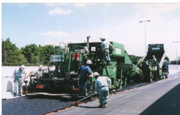
Photo 2: DL Pave construction situation
