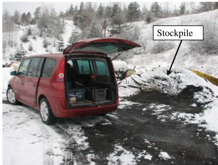
Figure 5: Stockpiled oil gravel made of bio road oil in Kouvola.
