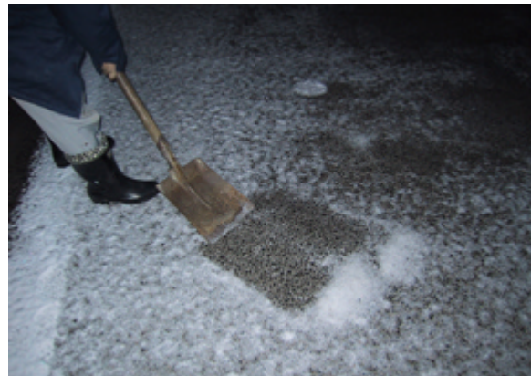
Photo 2: Condition of pavement after snow was removed
