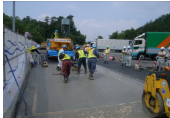
Photo 4: Pavement construction in parking area of Chugoku Highway
