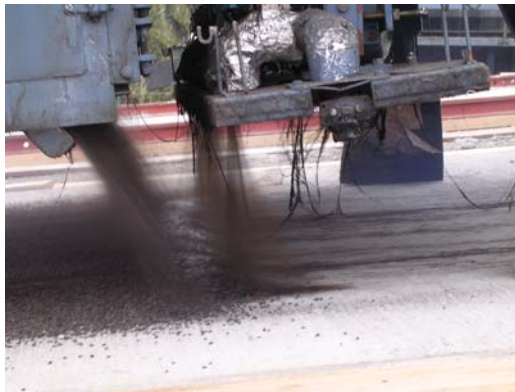
Figure 9: Spreading of foamed asphalt and precoated chips
