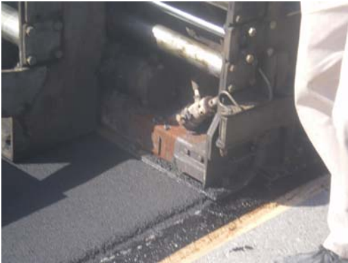
Figure 13: Application work (thickness of 10 mm)
