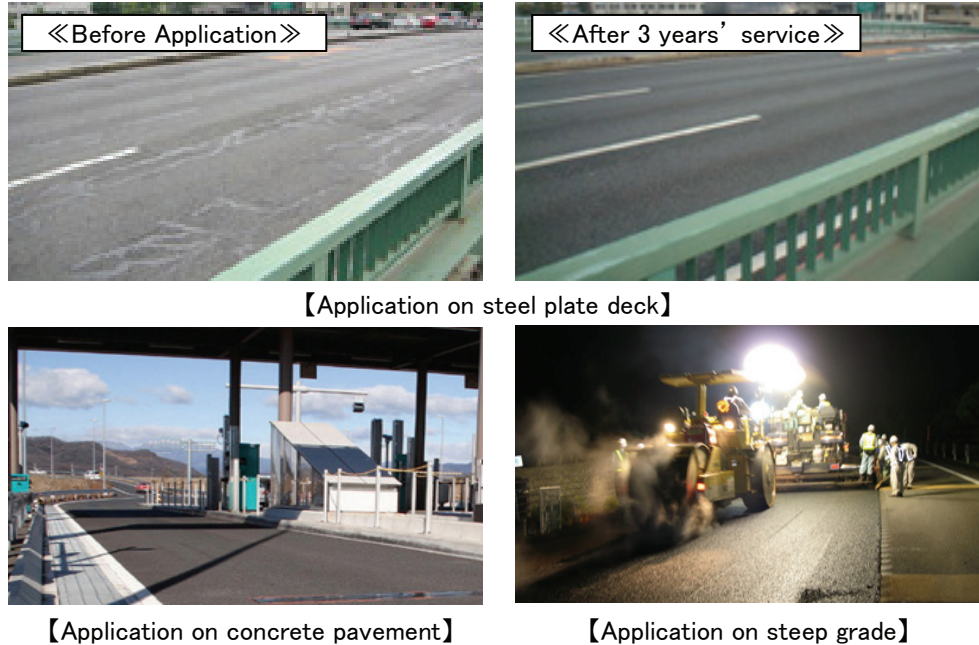
Photo1: Examples of installations under specific conditions
