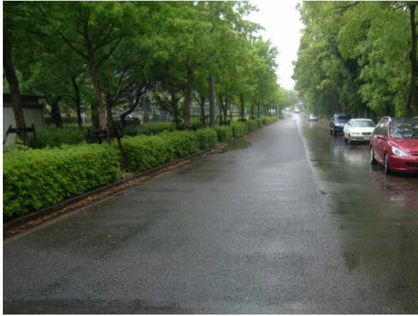
Figure 6 Road surface in 3.5 mm/h rain six years after pavement in 2001
