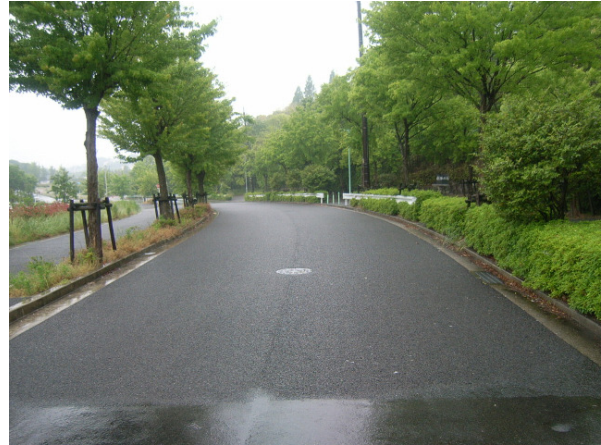
Figure 7 Road surface in 3.5 mm/h rain five years after pavement in 2002
