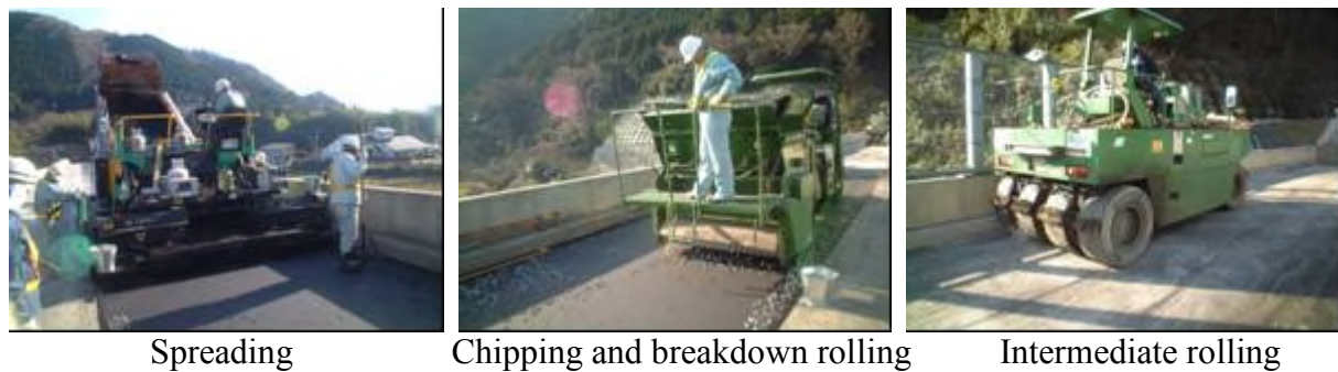
Photograph 2: Paving of Gum Rolled asphalt
