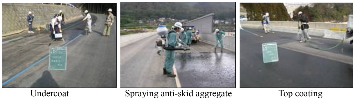
Photograph 3: Surface dressing using MMA resin
