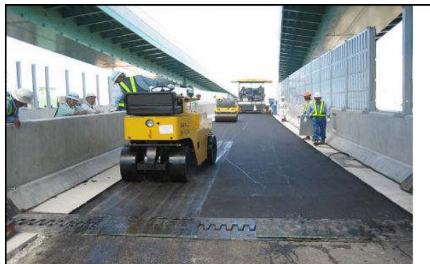
Figure 8: Rolling by a compact tire roller(3t)
