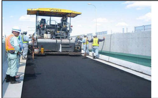
Figure 7: Spreading with 3.75m width
