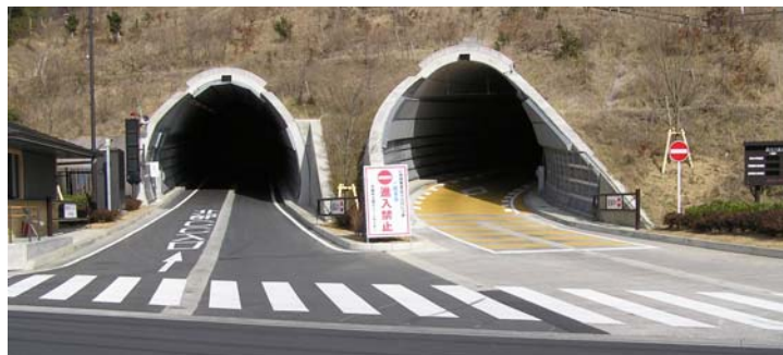
Photo 5: View of completed panel installation (left: entrance lane, right: exit lane) (Taken from near the property boundary)
