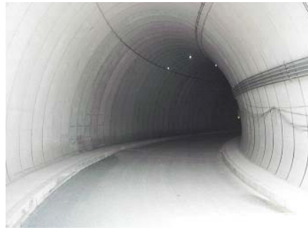
Photo 3: Before the installation of acoustic panels (exit lane)
