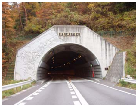
Photo 7: View of completed installation
