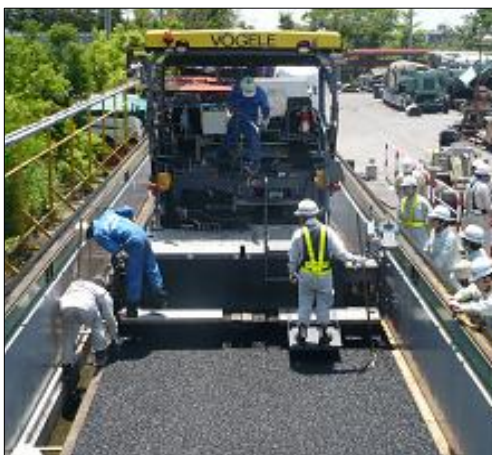
a) construction situation
