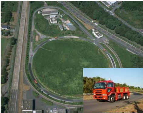
Photo1: Pavement Test Field and Loading Vehicle
