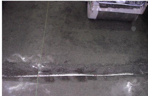
Photo 1 The establishment status to the top surface of the subgrade with FBG type strain gauge
