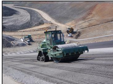
(Compaction by a self-climbing vibration roller)
