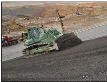
(Levelling by a bulldozer with a 3D-MC system)
