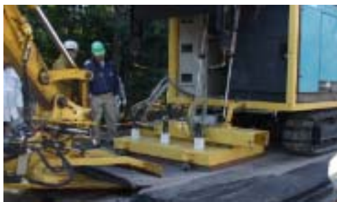
Photo 4: Test Construction Scene
