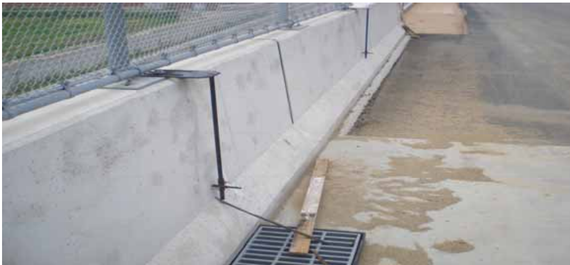
Photograph 2: Structure and jig on the railing
