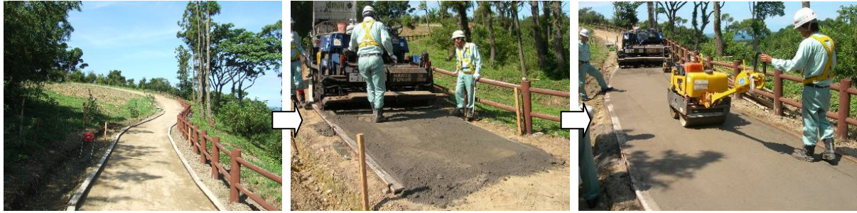
(1) Placing wood form
