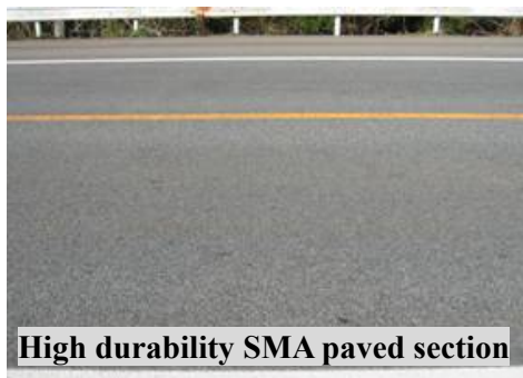
Photo 1: Road surface condition 47 months later the start of service
