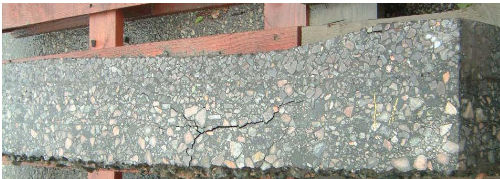
Figure 3: A beam was sawed from the slow lane showing significant deformation. (Cracking is from moving the beam and was not caused by traffic).
