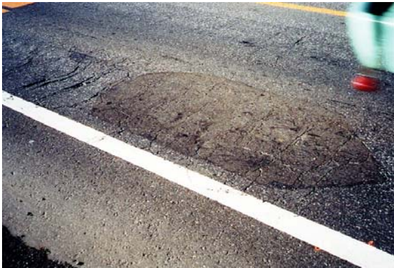
Photograph4: 9 months after repair
