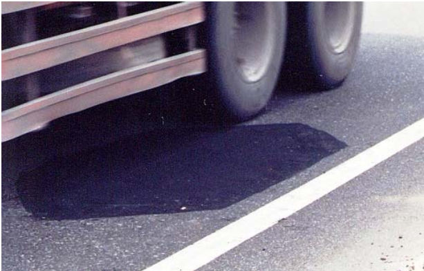
Photograph3: Traffic was opened immediately after repair
