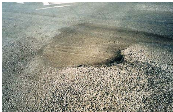
Photograph7: 9 months after repair
