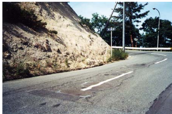
Photograph14: 3 months after repair
