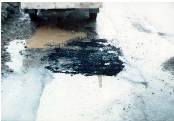
Photograph10: Traffic resumed right after repair
