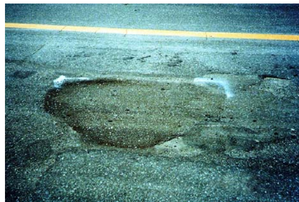
Photograph11: 3 months after repair
