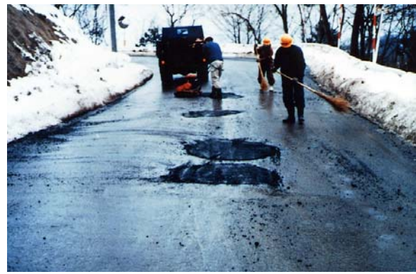
Photograph13: Scene of repair work
