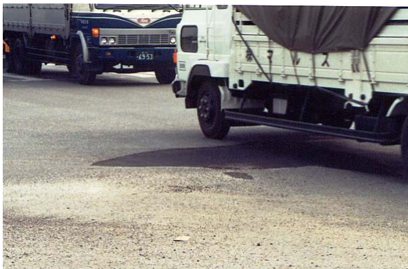
Photograph6: Traffic opened immediately after repair
