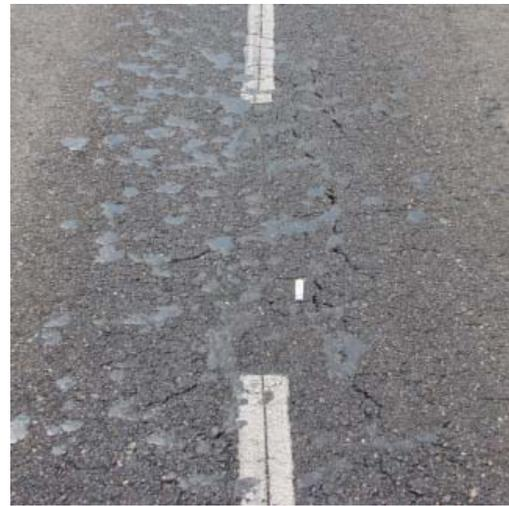
(b) Surface cracks with asphalt droplets on section 4-3B
