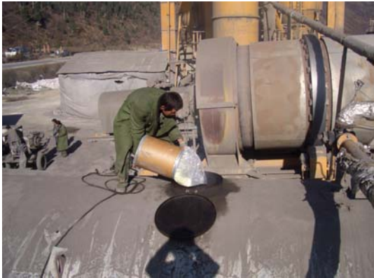
Figure 4: Adding additives into asphalt
