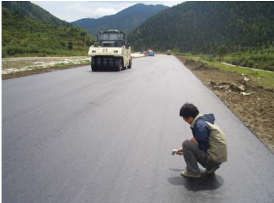
Figure 5: Roller compaction site
