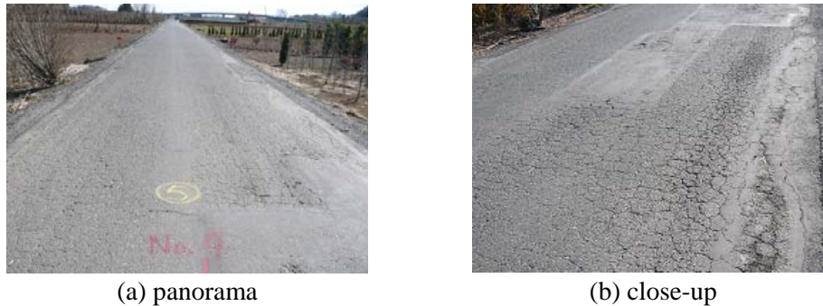
Figure 6: Typical surface condition ((a) panorama, (b) close-up).
