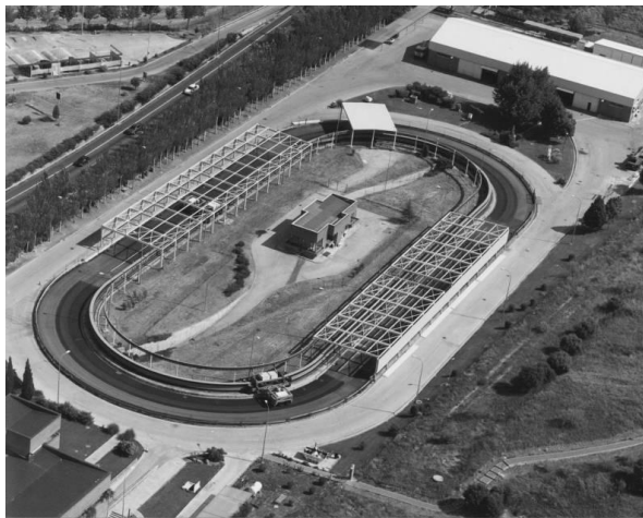
Figure 1 CEDEX full scale testing facility.
