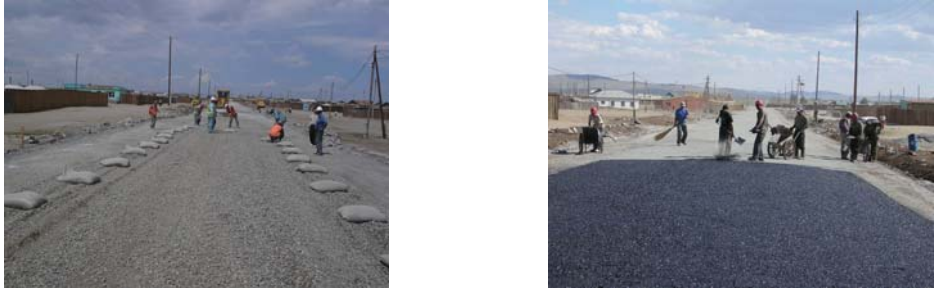
Figure 6: Labor intensive works in construction of CSTB and BST
