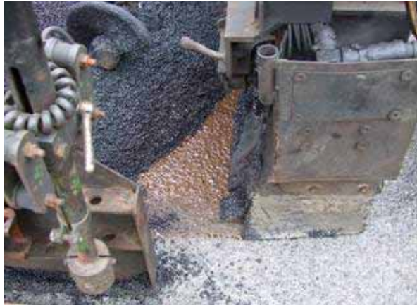
Picture-2 Emulsion spraying and
