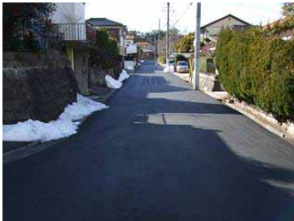
Picture-5 Road after construction
