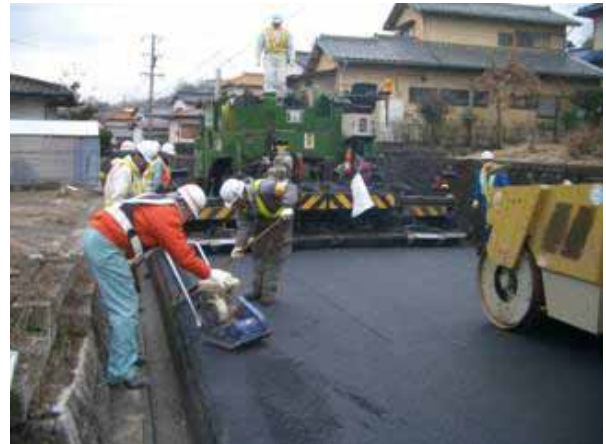
Picture-3 Spreading and rolling
