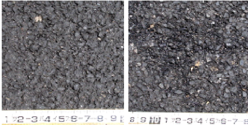
Picture-7 Macro photography of road surface
