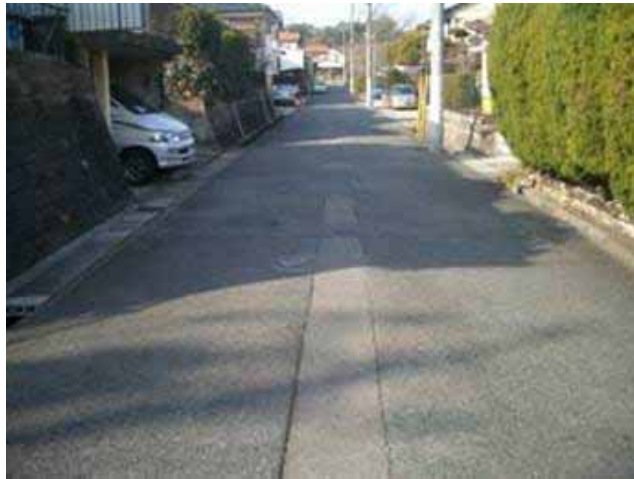
Picture-1 Existing road condition before construction
