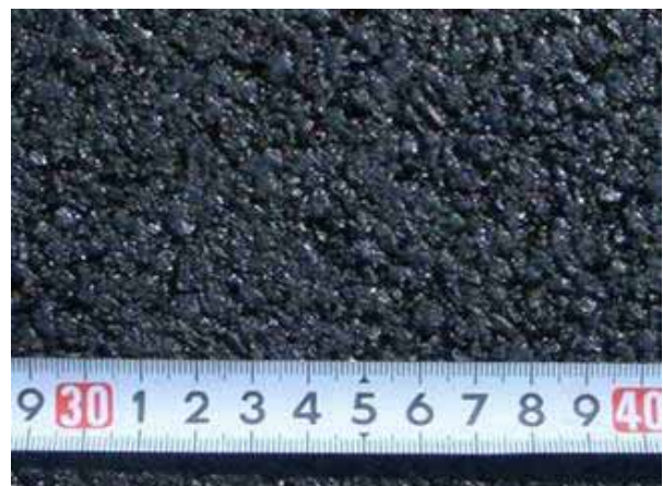
Picture-6 Finished surface after construction
