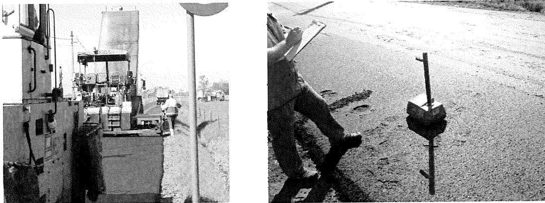
Figure 5: Paving of test tracks and nuclear density measurements during compaction
