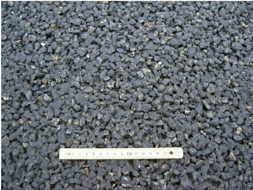
Photograph 1: Porous HMA pavements right after pavement
