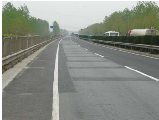
(a) Transverse Crack (Patching)
