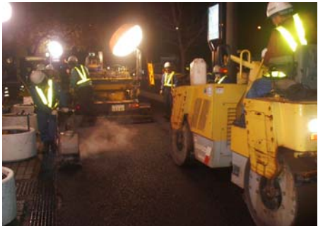
Photo 9: Laying of Surface Course (Rolling and Compacting)
