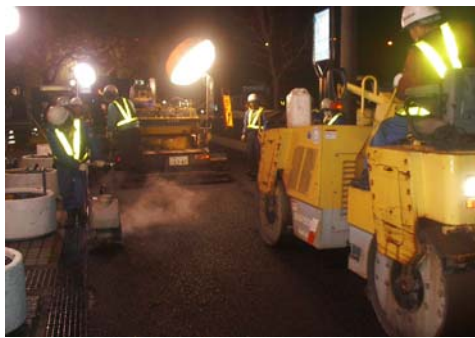
Photo 10: Water Jet Operation
