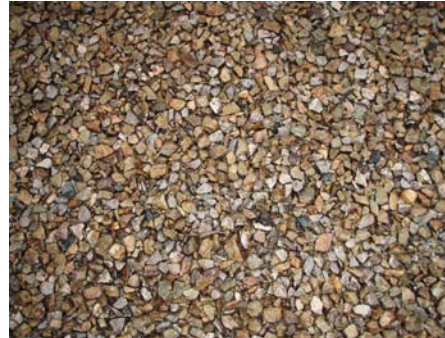
Photo 11: Exposure Condition of the Surface after the Water Jet Treatment
