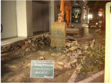
Photo 7: Removal Condition of the Previous Brick Blocks
