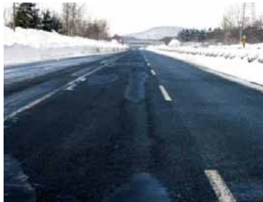
Photo 1: Scaling and abrasion in a snowy section
