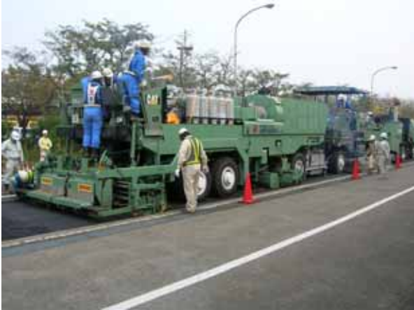
Photo 5: In-site surface recycling for the binder layer
