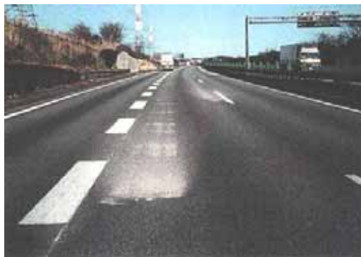
Photo 2: Particles blowing up from Porosity
