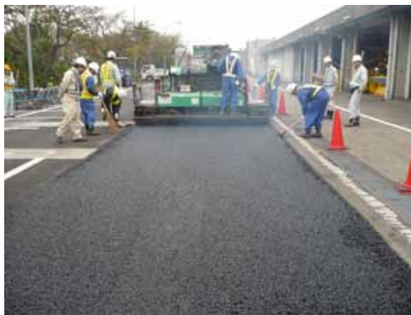
Photo 6: Finishing the recycled porous layer
