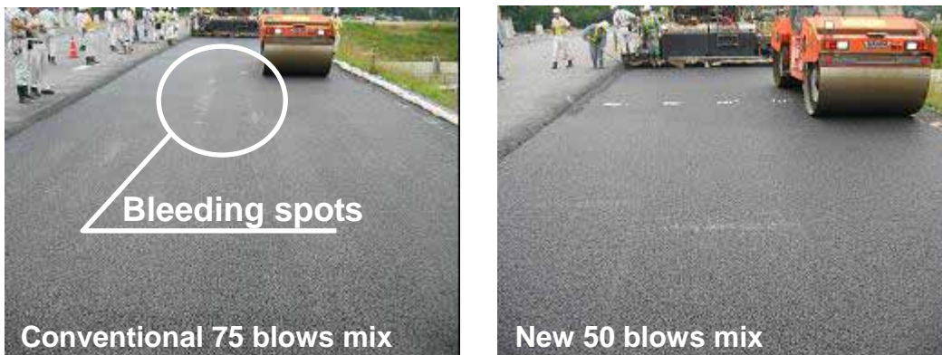
Photo 3: Comparison of road surface
