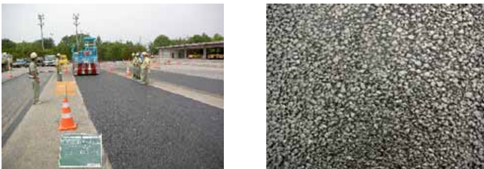
Figure 10: Satisfactory road surface as designed (Highly polymer modified asphalt, SBS 8%)
