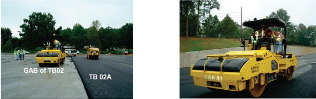
Figure 4: IC roller on GAB subbase (left), and HMA application (right)
