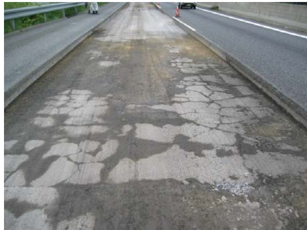
Photo 1: Cracking to granular base
