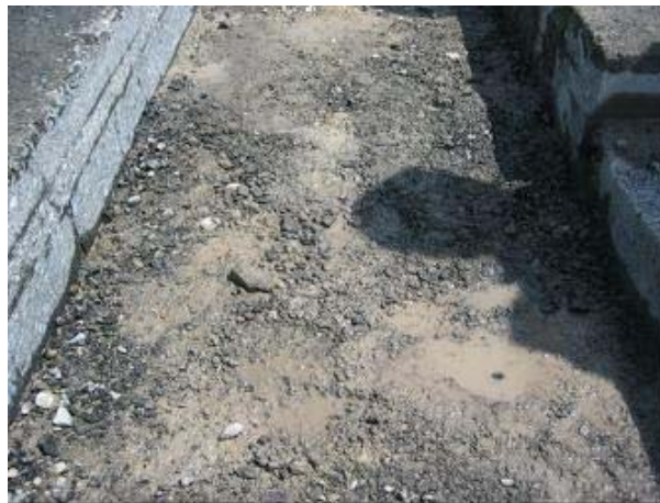
Photo 4: Water in granular base layer
