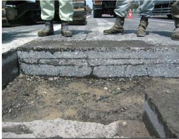
Photo 3: Cracks in bituminous layers
