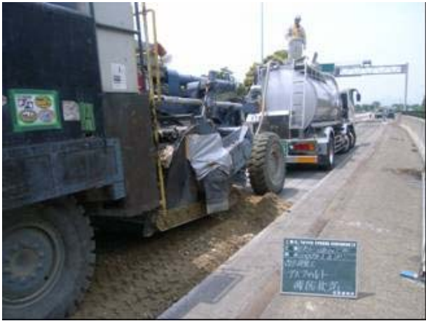
Photo 5: Ongoing Machinery with Foamed Asphalt
