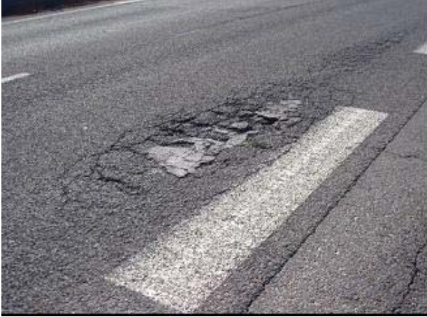
Photo 2: Potholes from porous asphalt
