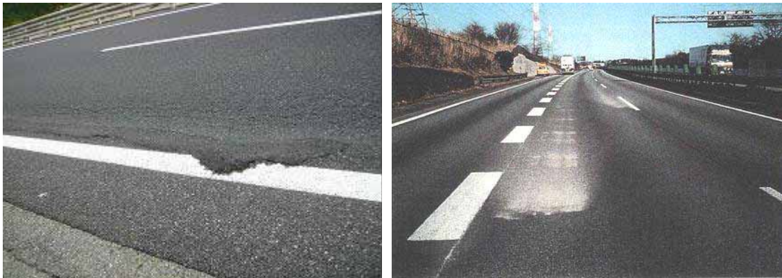
Photo 1: Partial plastic flow (left) and blowing up of particles from porosity (right)
