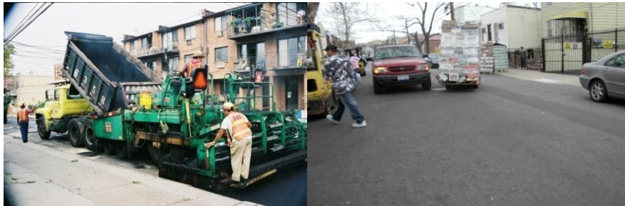
Figure 5: Photos during construction and after 7 years of service
