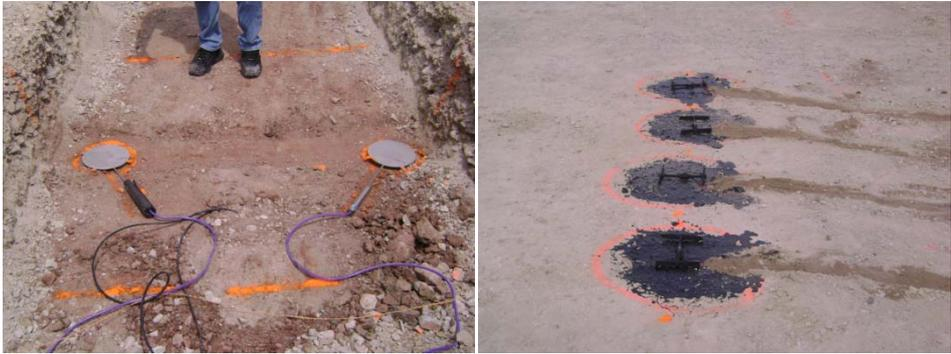
Figure 2: Installation of Pressure Gauges in Subgrade and Asphalt Gauges at the bottom of the RBM.
