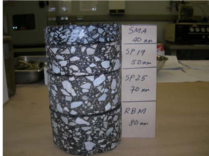
Figure 1 : Core extracted from completed main lanes of the RHVP showing position of RBM layer.
