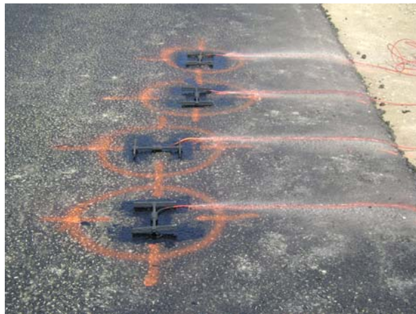
Figure 4: Longitudinal and transverse strain gauges installed in the RBM layer.
