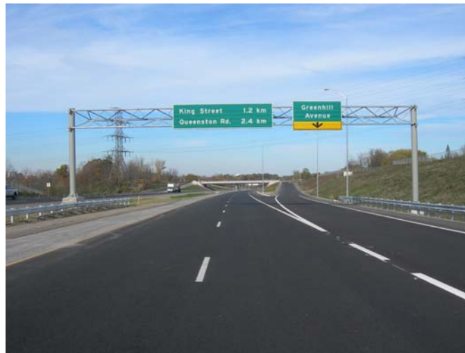
Figure 6: Completed section of RHVP.
