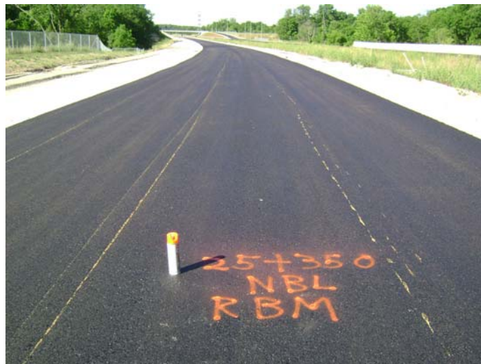
Figure 3: RBM layer after adjustments to the aggregate gradation.
