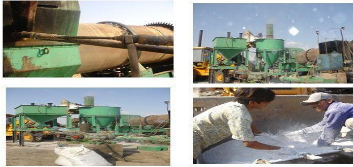
Photo 1: Distribution of Stabilizing Additive in Drum Mix Plant
