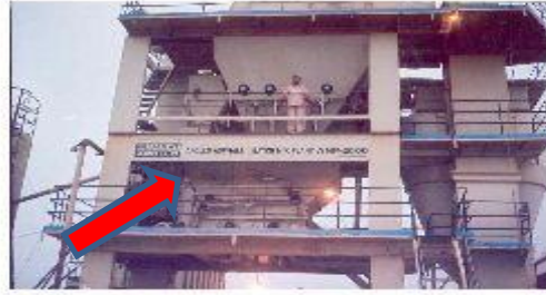
Photo 8: Aggregate Mixing Plant
